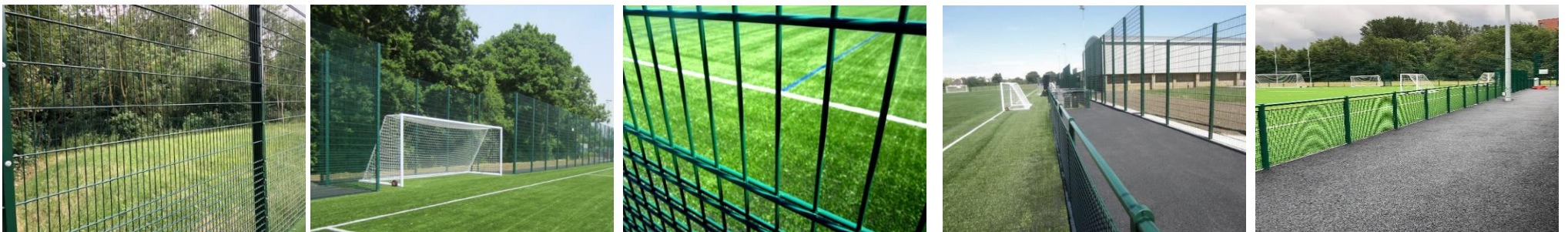
Rigid panel ballstop fencing to perimeter of facility, powder coated dark green to be discrete against a rural backdrop
